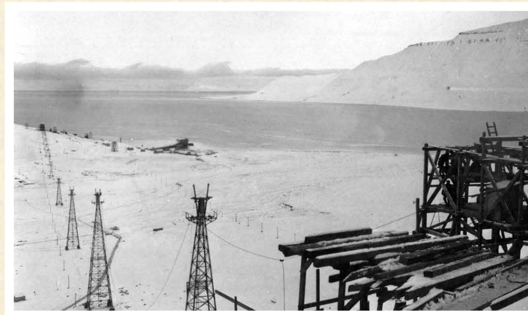
The cableway from Mine 2a <sup>4</sup> in 1921. The six nearest trestles are made of steel and were called towers.
