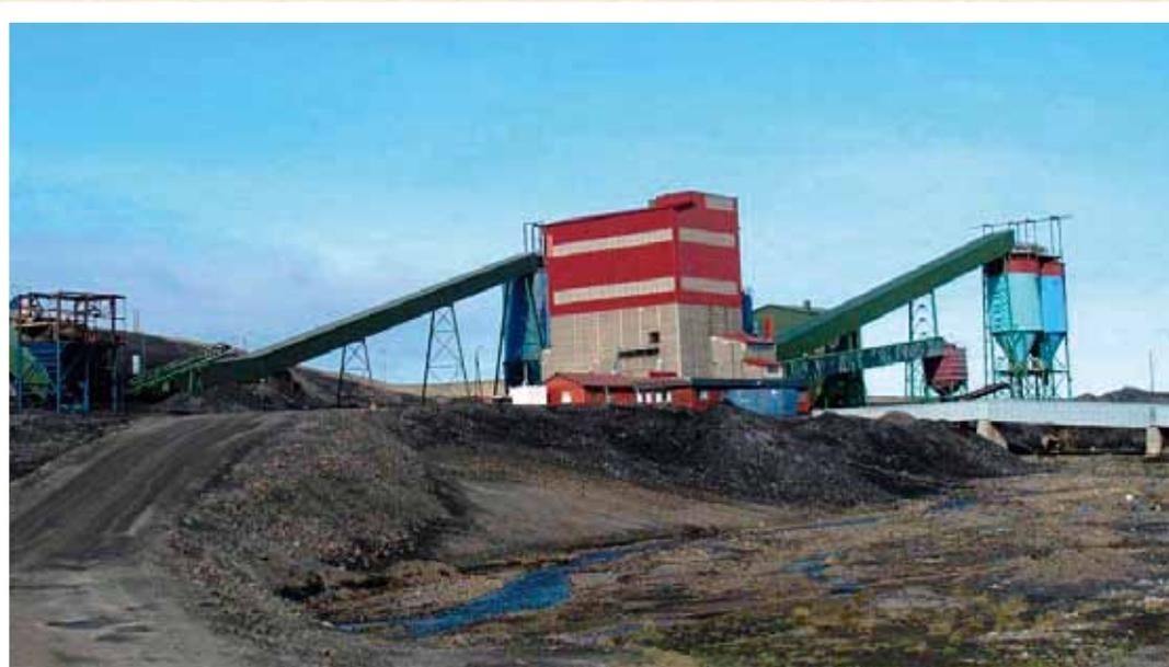
Cleaning and sorting plant, ORV in 2009 <sup>71</sup>. Built in 1954 and rebuilt several times. Separates out stones and sorts coal by size. Also called the preparing plant and the cleaning plant. It was also the site of SNSK's laboratory for analysing coal quality. Demolished in 2010. Photo: Per Kyrre Reymert
