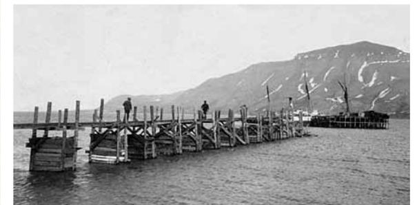
Old dock <sup>11</sup> under construction in the summer of 1907. There are goods on the dock even though the pier has not been completed.
