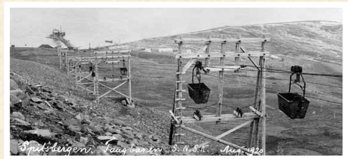
Longyearbyen's first cableway was built in 1906. It ran from Mine 1a, the American Mine, to the coal depot and then onwards to the loading dock on the left of the picture. This cableway was in operation until 1920. Photo SNSK.
